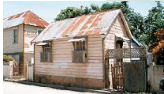
36a Cornwall Street, Falmouth, pre and post its restoration by Falmouth Heritage Renewal
