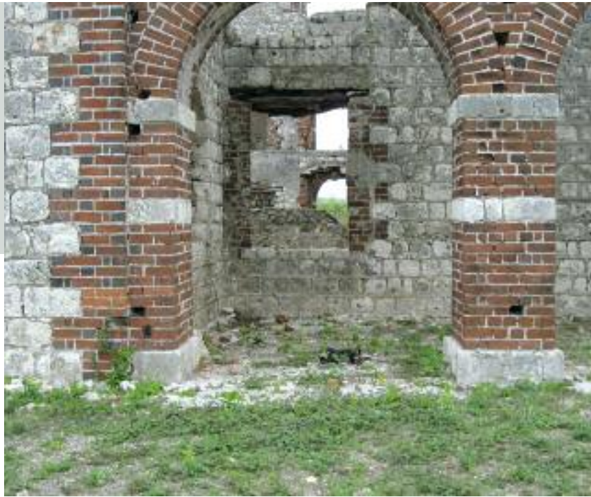
Right: Colbeck Castle. east elevation showing downspout fixing points
