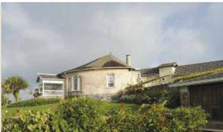
Tharp's last house, Jamaica's circular Chippenham Park
